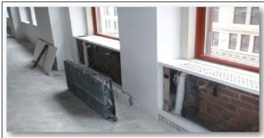
Figure 2-28: Empire state building windows; Embraced from (ESB, 2020)
